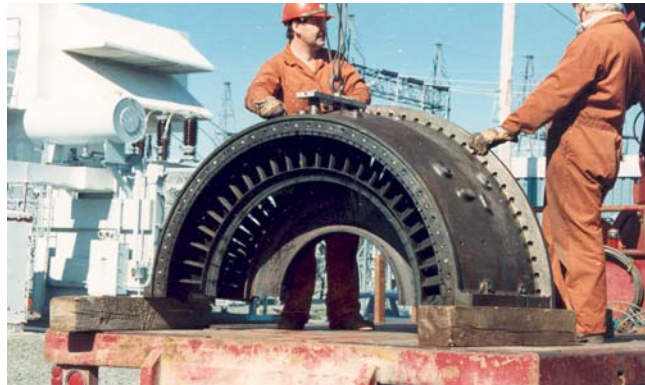
Old casing from a Cadillac gas turbine.
